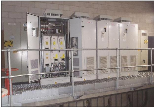
**Caption:** Yorkshire Water's Bradford Esholt wastewater treatment plant is saving over £61,000 on energy costs following the installation of ABB variable speed drives on its re-circulation pumps.
