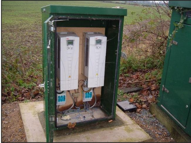
**Caption:** ABB low voltage AC drives installed at rural pumping stations are saving Yorkshire Water the cost of installing three-phase supplies at remote sites.
