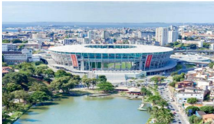
Arena Fonte Nova 18 x ZX0.2 Panels for the WM station
