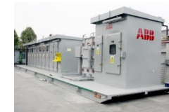
Package #2 - Outdoor skid medium voltage connection
