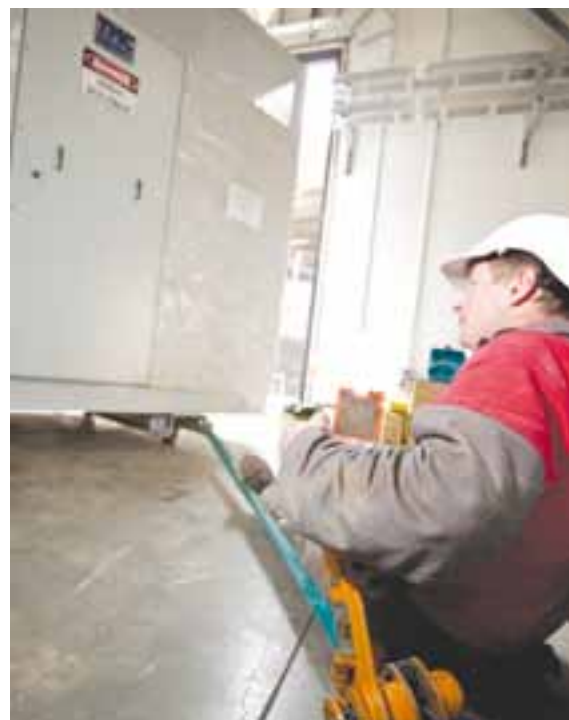
ABB's Aaron Emerson winches the transformer into place.
