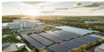
Reducing emissions in industries ABB Ludenscheid factory, Germany
