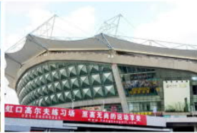
ABB Ability™ EDCS in football stadium Buildings Shanghai's Hongkou
