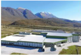
ABB Ability™ EDCS in cold storage facility Pacaro Logistic
