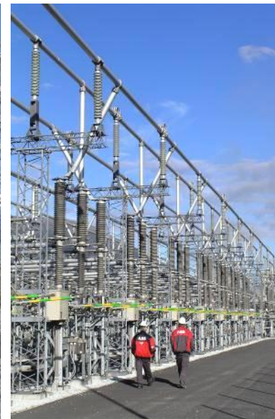
Disconnecting Circuit Breakers
