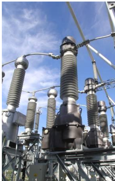
Instrument Transformers
