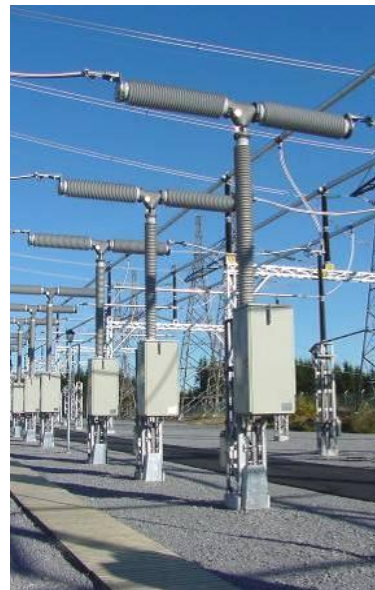
Live Tank Circuit Breakers
