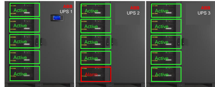
Status 2: Module operating modes when a fault with module has been detected
