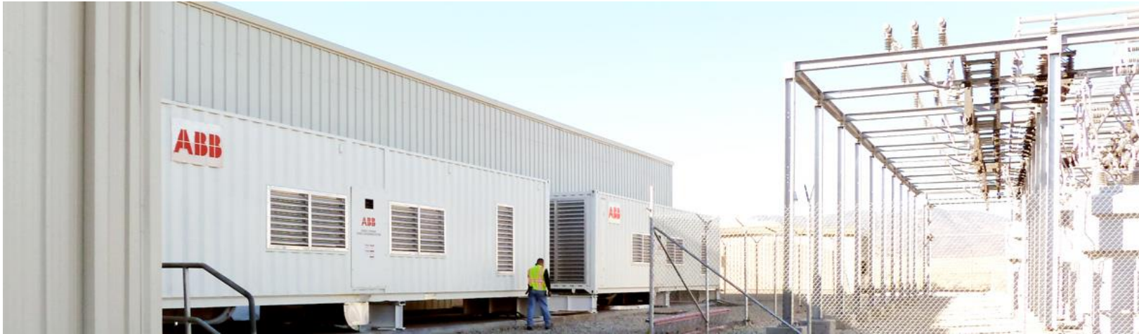
8 MW / 32 MWh Tehachapi Storage Project
