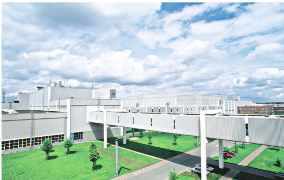
Mercedes-Benz in Rastatt: Third cogeneration plant commissioned.
