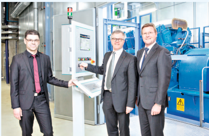
Cogeneration plant commissioning in May 2013: From left to right: Rolf Busch (project owner), Hans Jürgen Pütsch (mayor of Rastatt) and Peter Wesp (head of plant).
