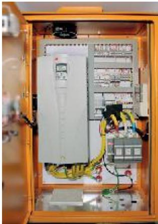
3. One of the ABB drives installed at the pumping station.
